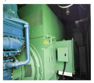
Complete Genset Control and Protection system with a local control panel located in the generator unit and a remote-control panel in the sub-station with an interface between the two, with connectivity with the SCADA system of the site was manufactured in house by PI. This system includes high end parameters for control, complex operation philosophy based on site requirement, High end protections with redundant serial communication and complete controls over the generator unit.
